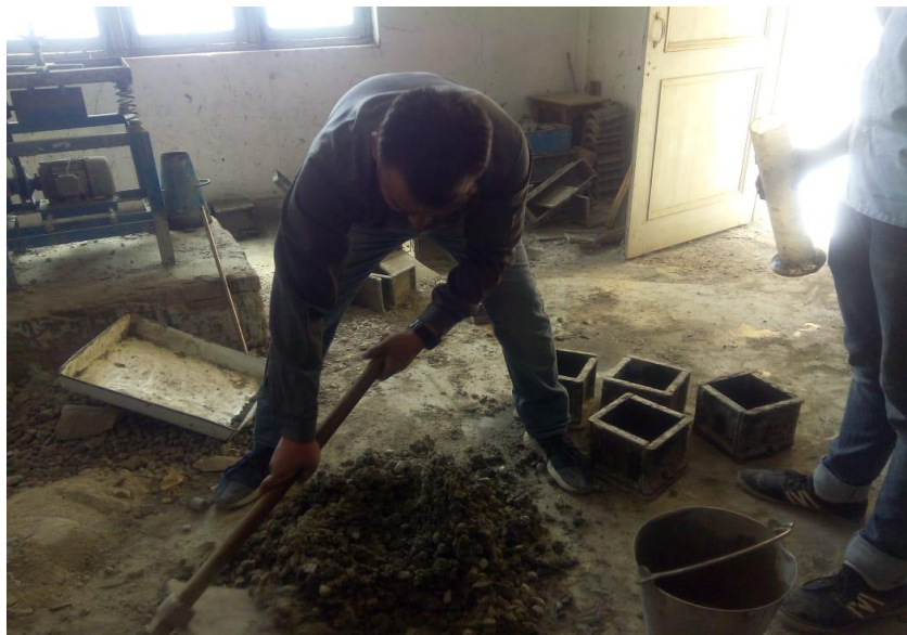
Fig. 3.1 mixing of concrete
